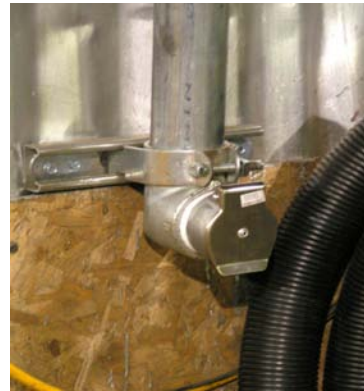
Inlet Valve shown installed in 90-degree adaptor elbow
