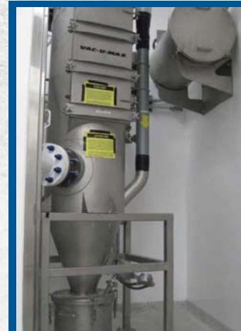
VAC-U-MAX Central Vacuum with Chemical Suppression HEPA2
