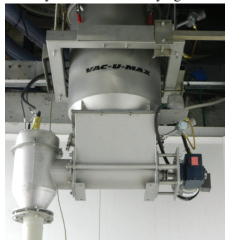
VAC-U-MAX dedicated vacuum receiver for loading 55 lb bags.
