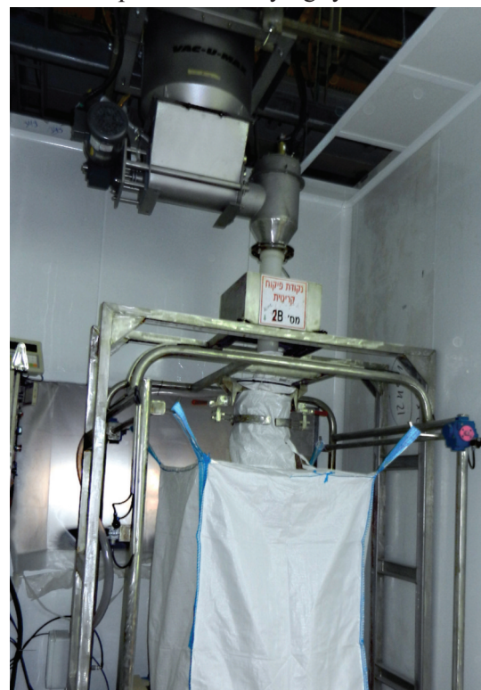
VAC-U-MAX vacuum receiver above 2,000 pound super sack.
