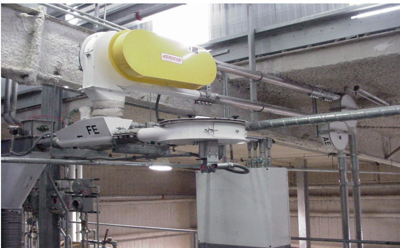
Transfer Point Between Type 450V and 250H Aero-Conveyors.
